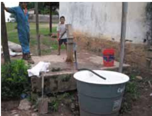
Pump for groundwater and source water tank
